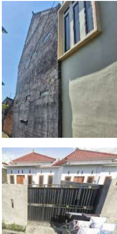
Figure 6. Representative examples of adjacent residential buildings exhibiting pounding potential due to insufficient separation distance
