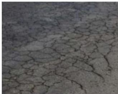
Gambar 1 : Alligator Cracking
