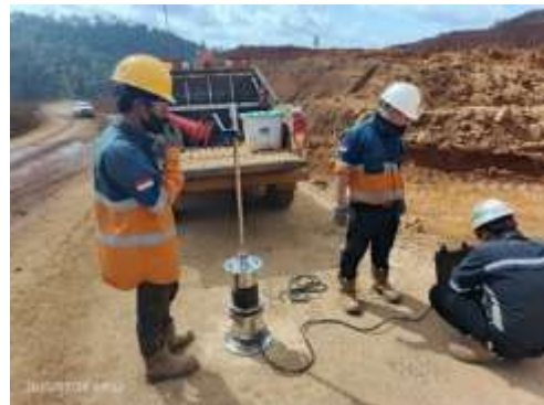
Figure 2. Light Weight Deflectometer Test
